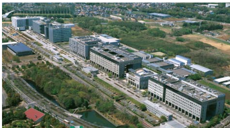
The center building is ISSP.
